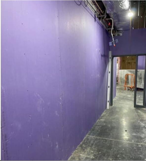
Interior drywall progress
