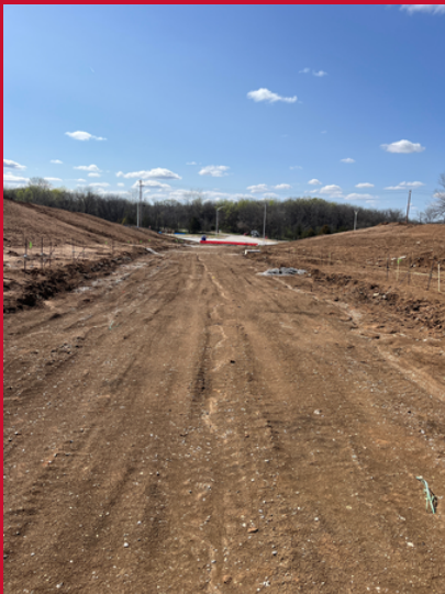
Road prepped for subgrade and asphalt activities to begin
