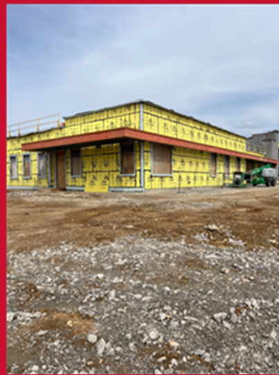
Air barrier detailing ongoing
