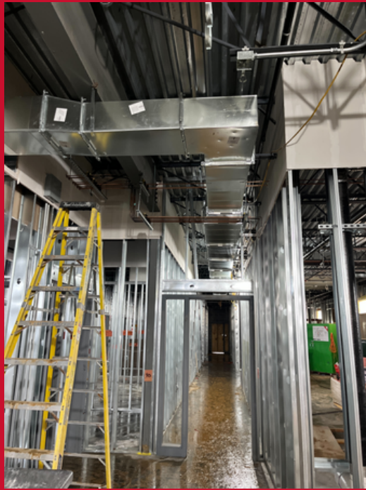
MEP interior installation ongoing
