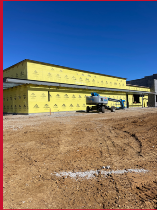
Completed exterior framing, sheathing and parapet caps
