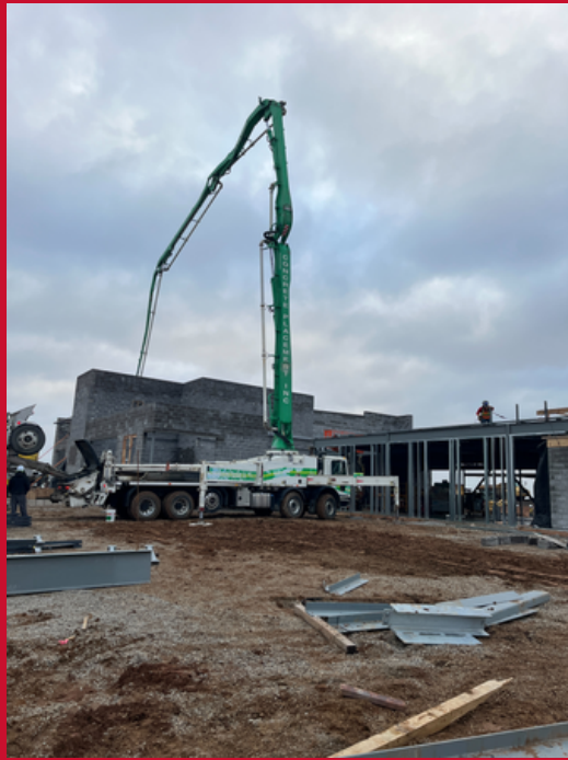
Concrete pumping at the elevated decks
