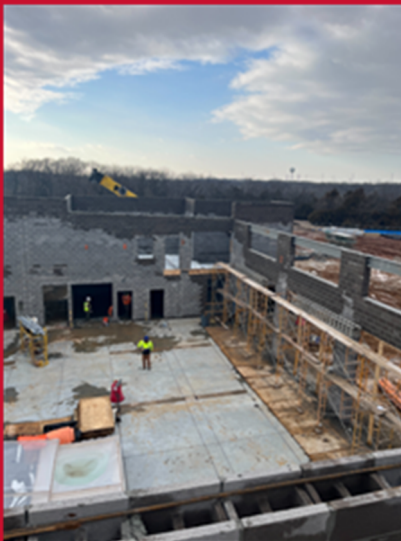
Apparatus Bay Topped Out and Ready for Bar Joists
