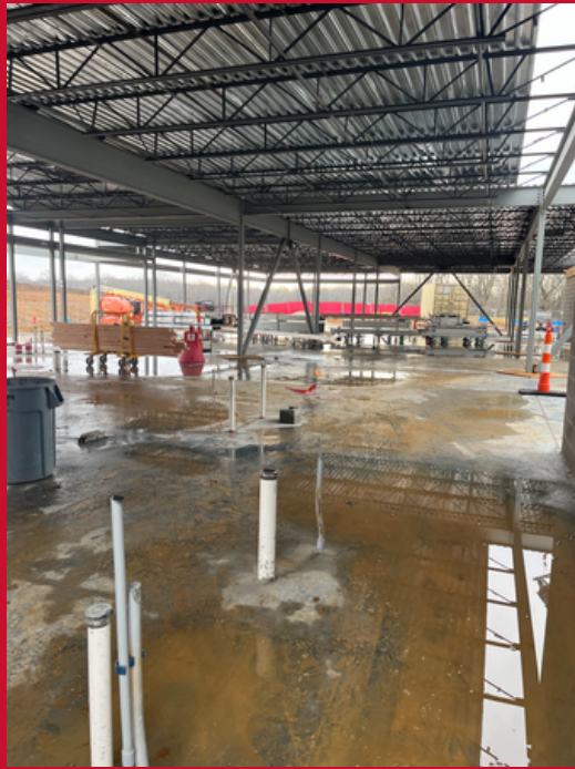
Structural Steel, Bar Joists and Decking at the Living Quarters
