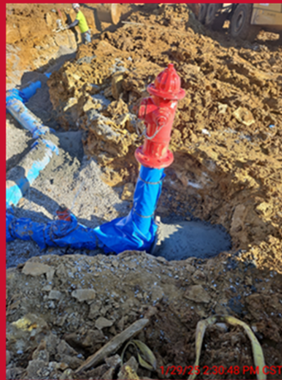
Water Main Installation Complete to Fire Hydrant at South Side of Building
