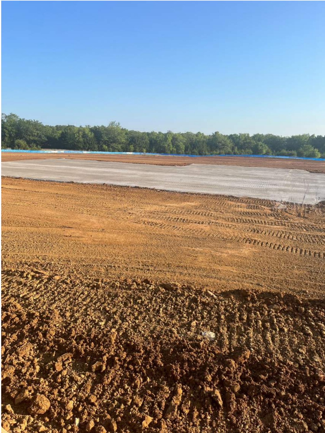
Fire Station Pad ready for footings
