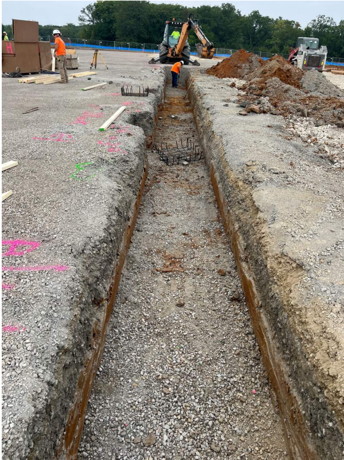
First footing dig at NE corner of building pad in app bay
