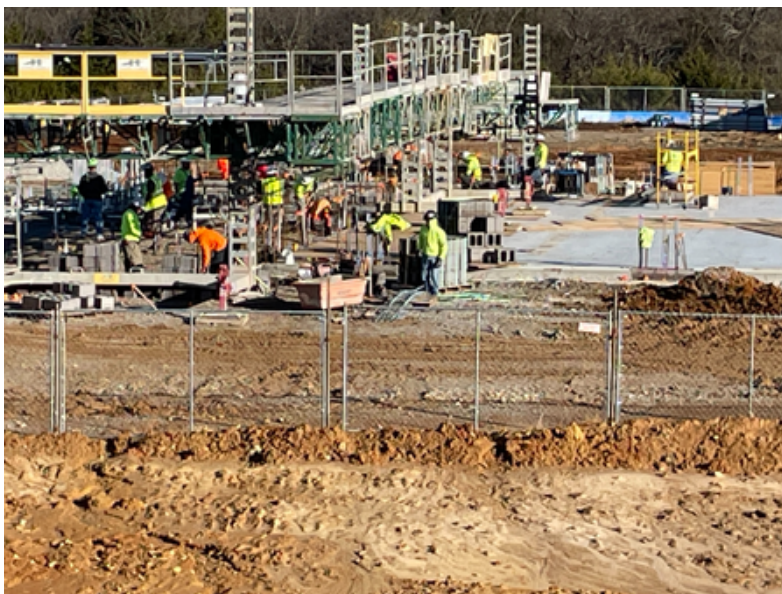
Hydro scaffold in place, first sections of CMU being installed West wall of app bay 11/15
