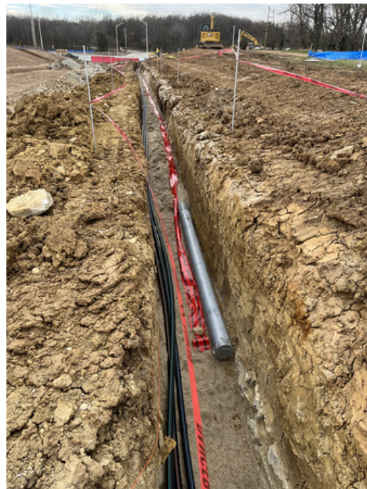
Electrical/fiber underground along North side of 102 nd Street 11/26
